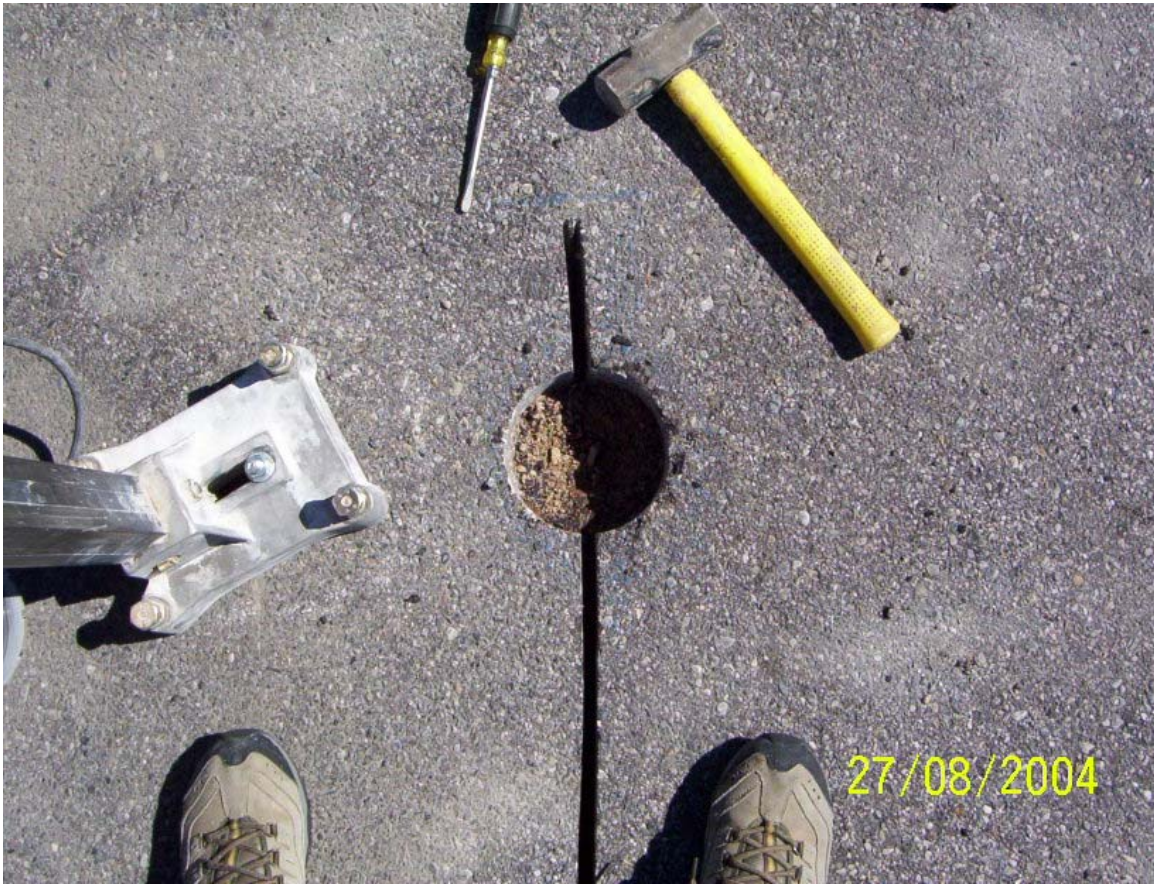
Figure 3-1. Core cut for the road sensor.
