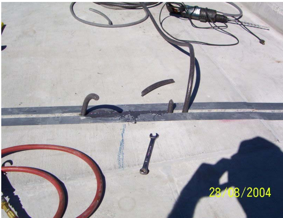
Figure 3-9. Backer rod is used as a dam to control the epoxy. Different epoxies can be used for directly around the sensor and along the cable. Since the epoxy used is liquid, the backer rod is used to dam the epoxy until cured.
