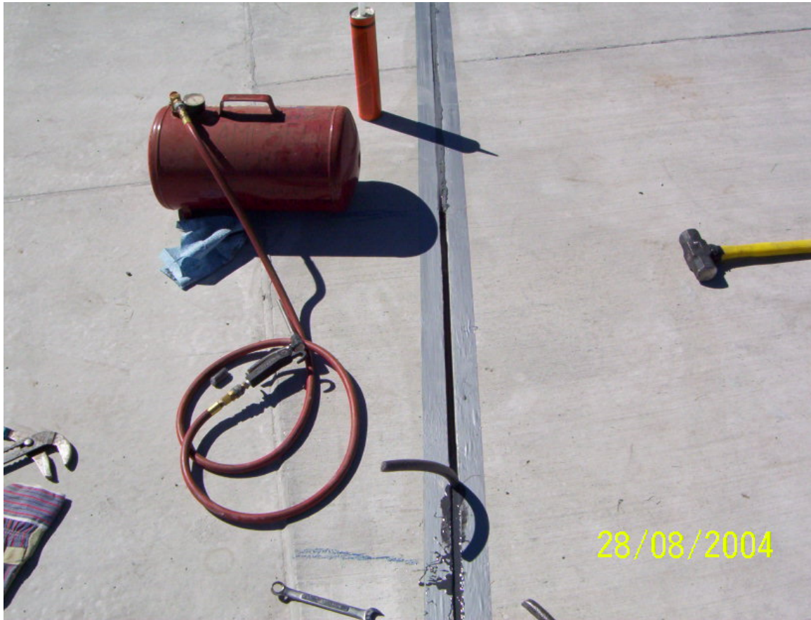
Figure 3-10. Compressed air is used to dry and clean the saw cut.
