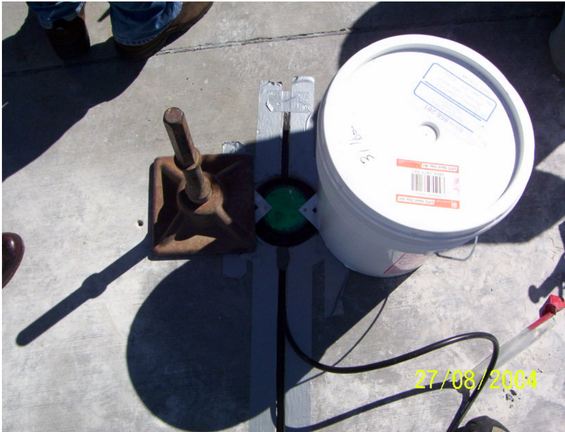
Figure 3-5. Weights are placed onto the levelling fixtures for the road sensor.
