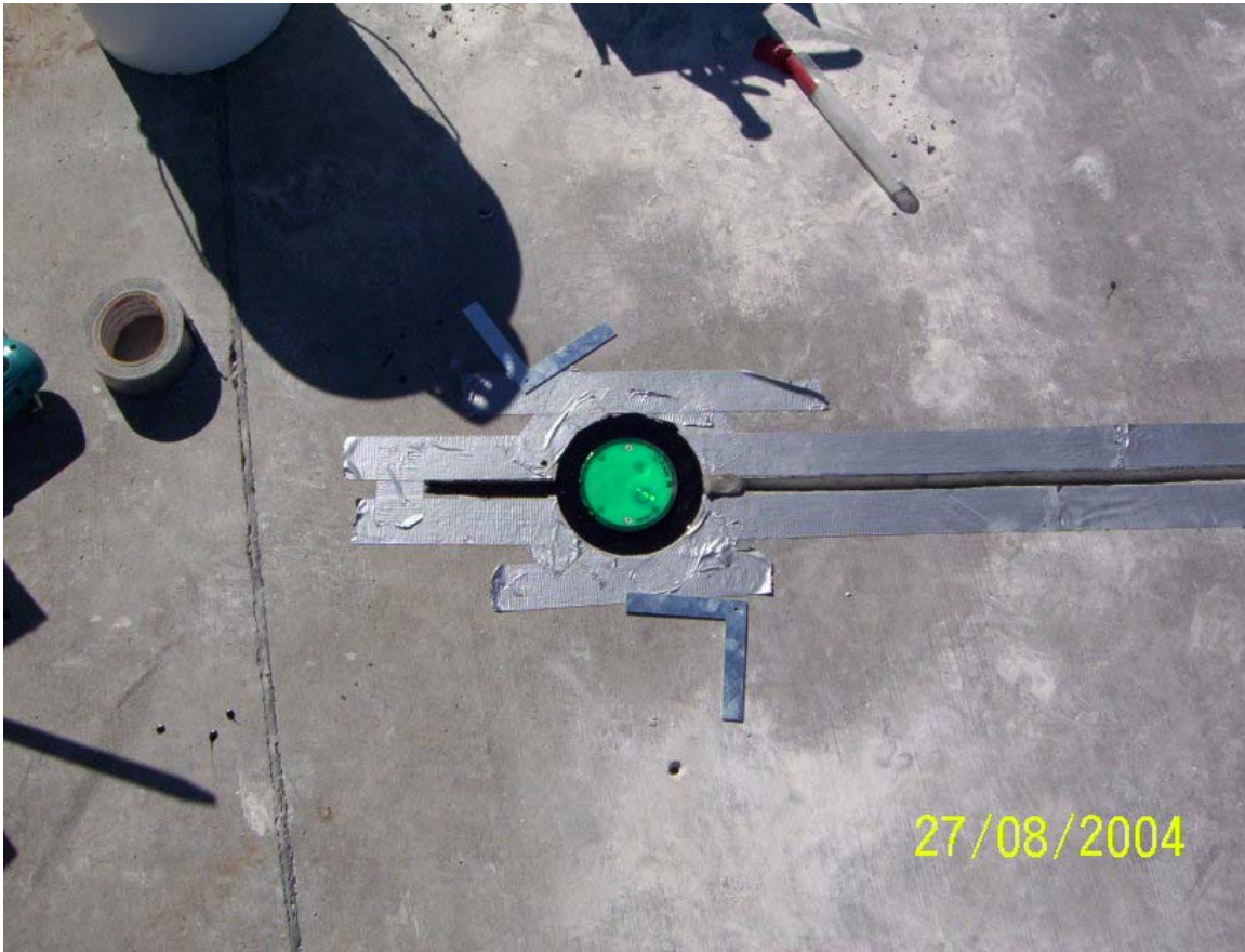
Figure 3-12. Finished epoxy application.
