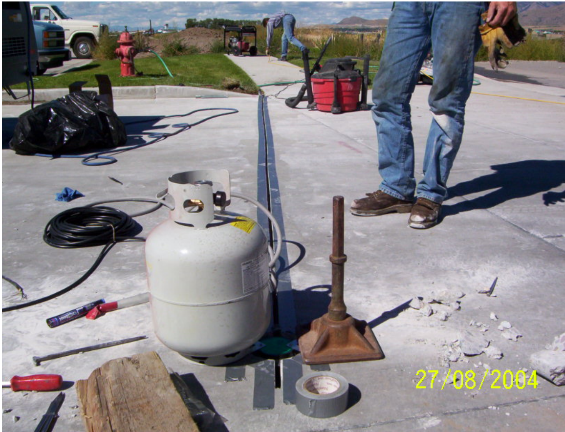
Figure 3-3. Saw cut is masked to control the epoxies.
