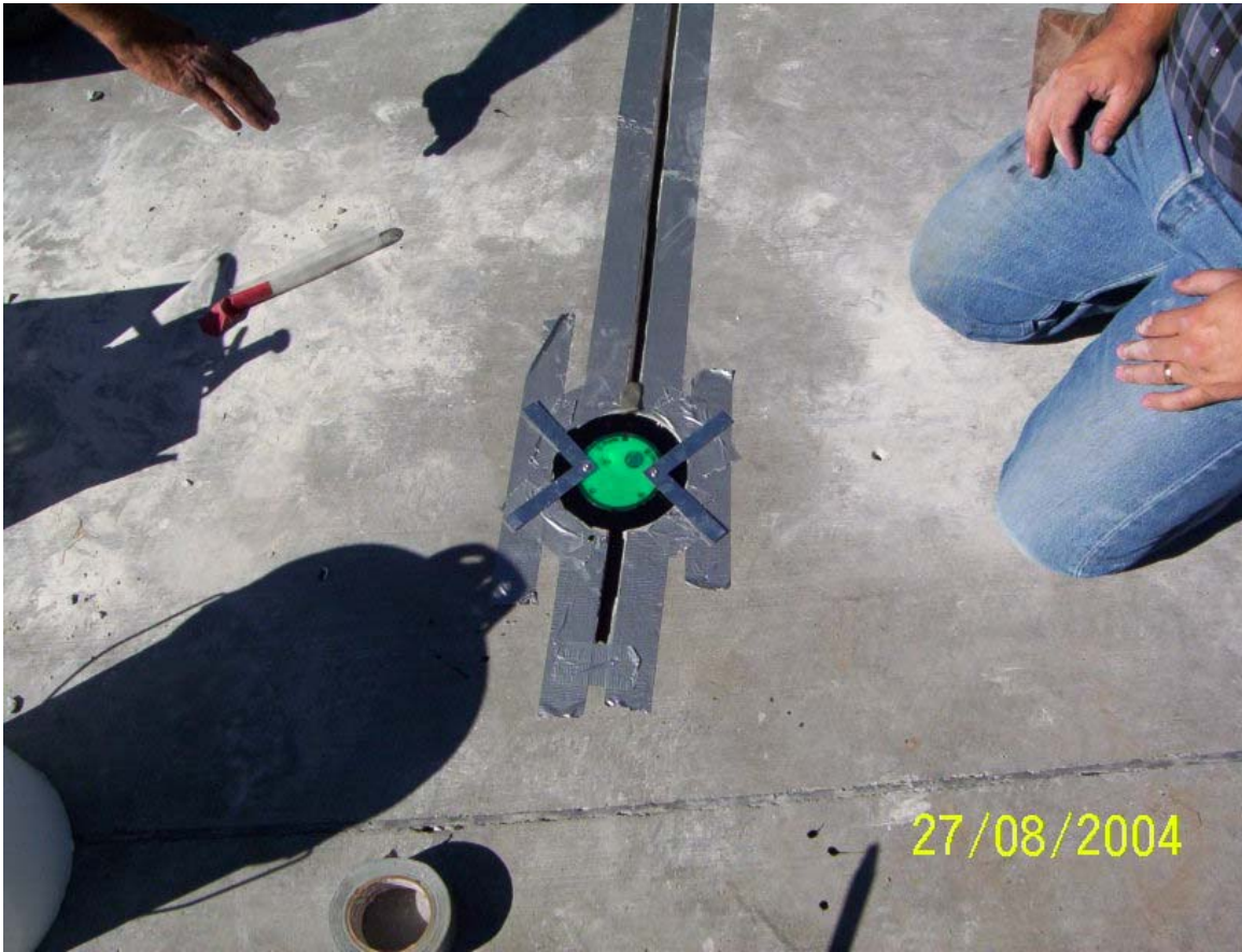
Figure 3-7. Finished pour, with weights removed.
