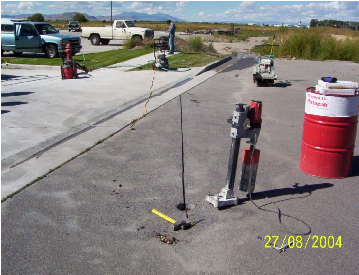
Figure 3-2. Core drill and saw cutting equipment.
