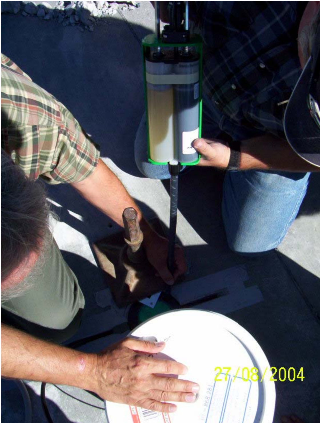
Figure 3-6. First pour of Fabick epoxy, (fast set), useable between 20° to 180°F.
